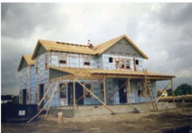
Photograph 4: Vapor Closed Exterior Continuous Insulation - If you used a vapor closed exterior continuous insulation like extruded polystyrene drying to the exterior was not possible.
