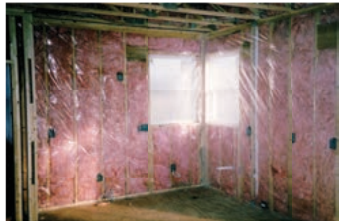
Photograph 2: Polyethylene Vapor Barrier – a "classic" Class I vapor retarder. Also a pretty darn good air control layer when installed with fastidious care...
