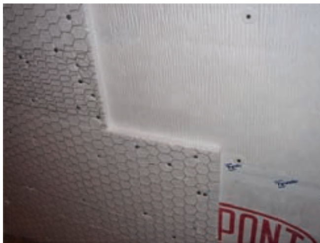
Photograph 6: Textured Building Papers - Placing the continuous insulation over textured building papers to facilitate drainage also provides redistribution of moisture.
