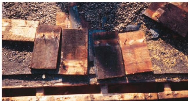
**Photograph 9: Damaged Decking**—The proof of the insulating is in the opening (old insulation contractor proverb). The deck did not stand a chance. Don't do this.
