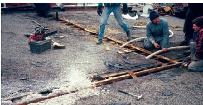
**Photograph 8: Flat Roof Being Dense Packed**—The roof is opened up and cellulose is being blown into the roof cavity dense packing it. The guy in the middle is Jim Fitzgerald, the absolute best guy in the world, and he could not make it work consistently. Does that tell you something, or what?
