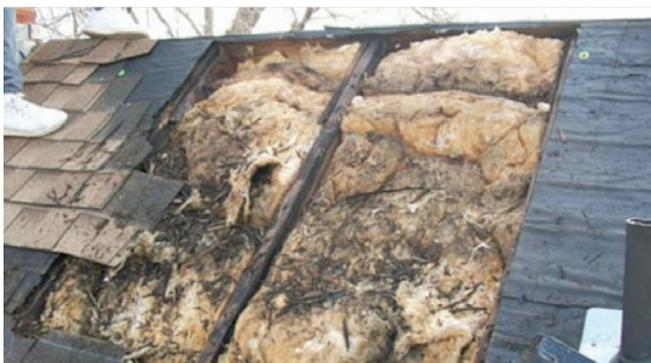
**Photograph 6: Unvented Cathedral Ceiling**—No one argues that it is a dumb idea to shove a bunch of fiberglass batts into a cathedral ceiling with no provision for ventilation air to remove some moisture. The results are often catastrophic.
