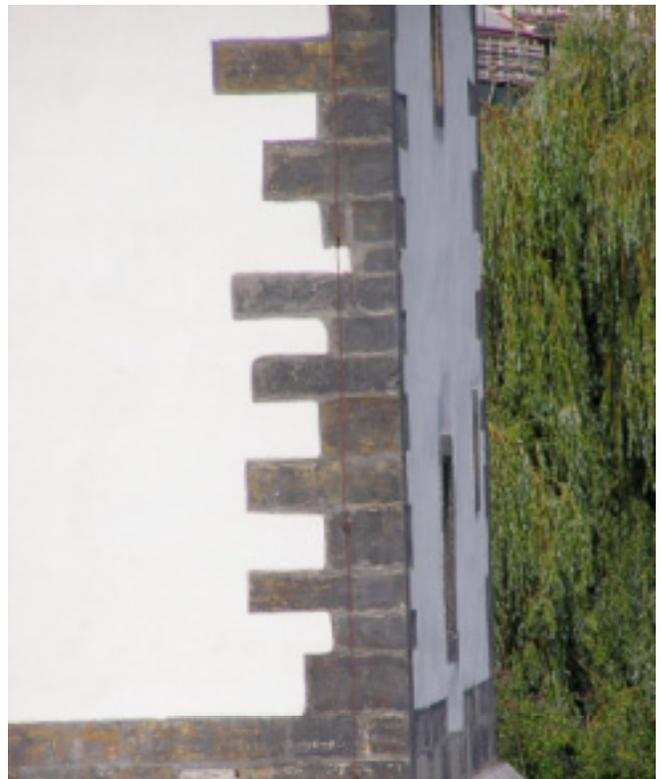
**Photograph 3: “Traditional Stucco”**—A protective layer of white stucco applied to a stone-rubble wall. The stucco was typically applied principally to the rubble “infill” between the quoins. Eventually even the quoins got stuccoed and the original function of the quoin was lost and quoins became aesthetic rather than functional.
