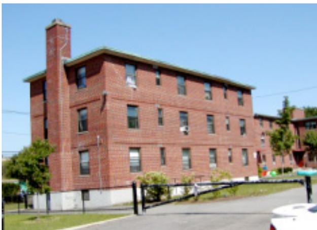
**Photograph 5: Face Lift Needed**—Uninsulated mass wall in Boston that is leaking rain, is cold, is uncomfortable, is an energy pig and is ugly to boot.
