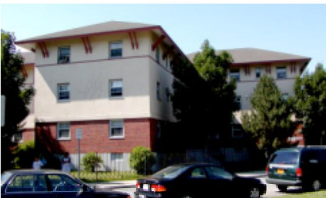
**Photograph 6: Saving A Building**—Add over hangs, a pitched and vented roof, and a “stucco screen.”
