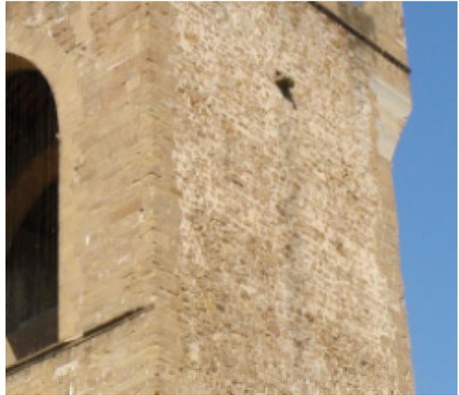
**Photograph 2: Quoin Assemblies**—Good stone corners and good stone lined “punched” openings with rubble comprising the “in-fill” of the wall.
