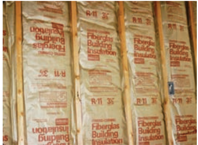
Photograph 3: Kraft-Faced Fiberglass Batts - The typical Class II vapor retarder was (and still is) a kraft faced fiberglass batt. The Class II vapor retarder allows inward drying in the summer time.
