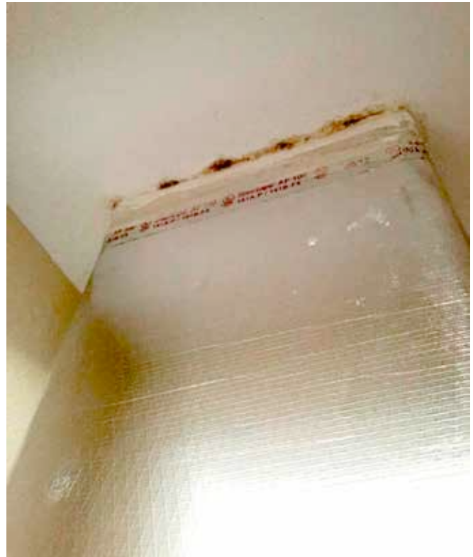
Photograph 7: Mold at Ceiling of Mechanical Closet —If all you do is put the air handler inside the house in a closet inside the house you will get mold. Not a lot. But some. It typically ends up at the ceiling of the closet where the supply plenum penetrates the ceiling. This problem goes away with a grille on the return plenum (see Figure 1 again) coupled with a jump duct or transfer grille.
